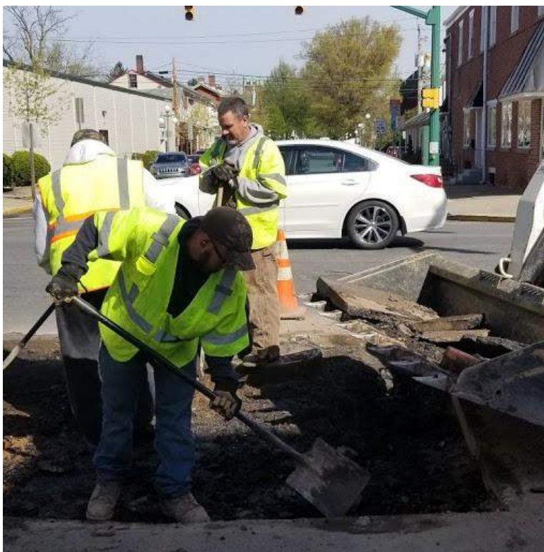
Collapsed manhole repairs, due to heavy vehicles, Market & Third Streets, Spring 2019.
