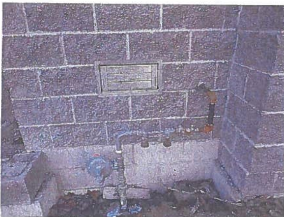
Engineered Flood Vent x 8
